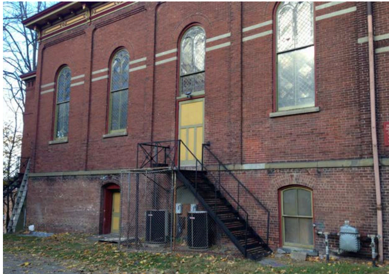
Figure 2.5 Vassar Institute side brick detail, lower brick portion (the faded part) is the original from Vassar's brewery (George, 2013).
